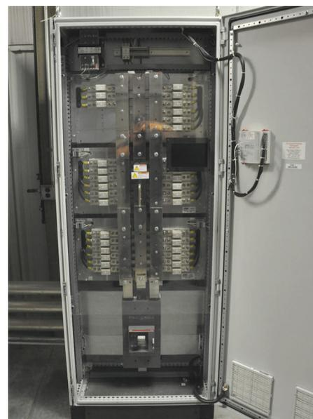
**StacoVAR Automatic Power Controller at the manufacturing facility**
